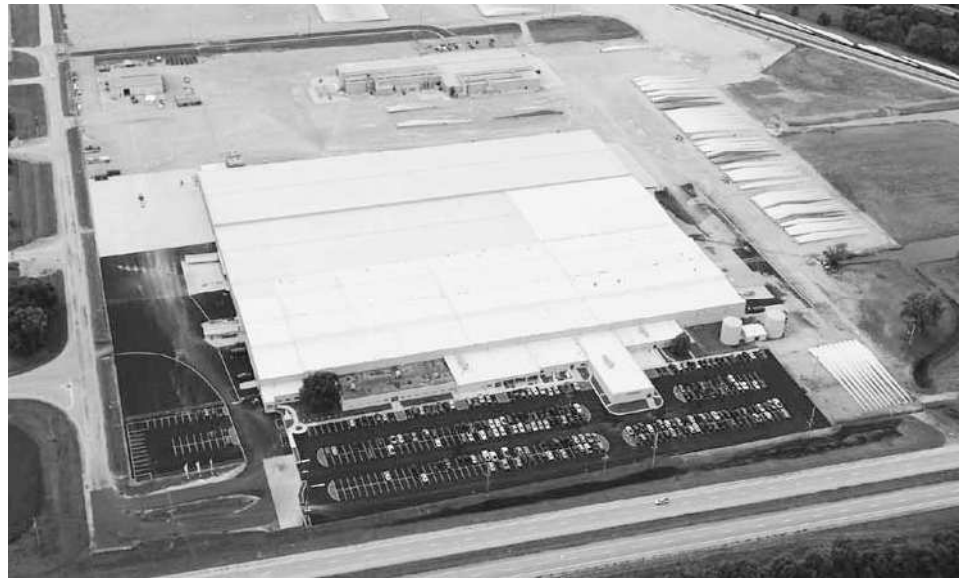
This $32 million Siemens Expansion Project required creative thinking and consistent communication by CCI and the building team to meet the extreme fast-track schedule and unique owner requirements.
