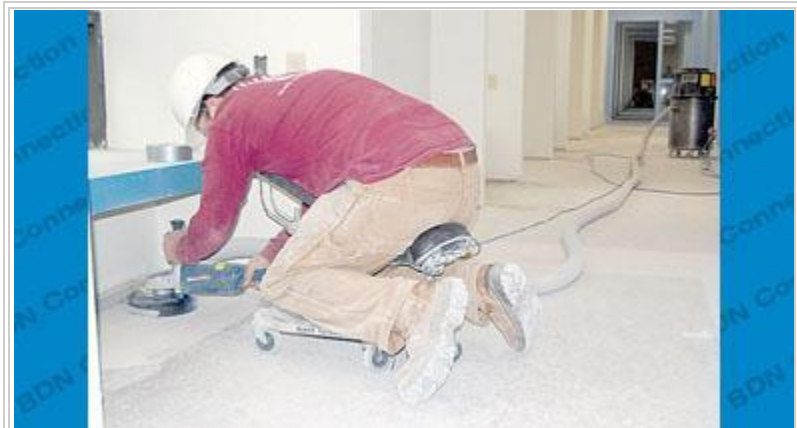
CCI worker Trent Austin polishes the floor at the former Beloit Library. The building renovations will be completed by July 2. Staff photo by Hillary Gavan
